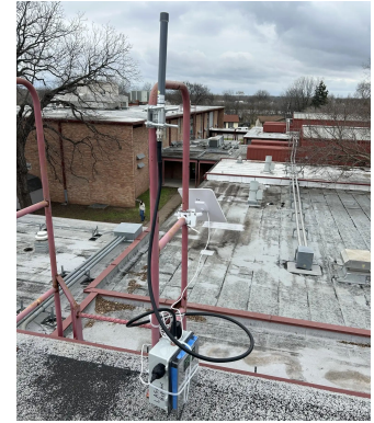
Clamped to an access ladder
